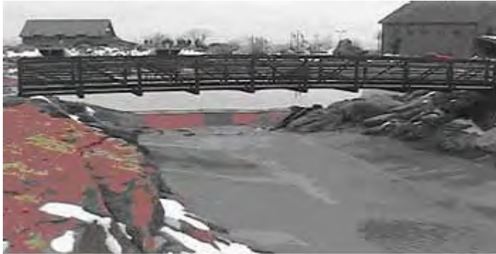
Upstream view of the first drop next to the observation bridge without water.
