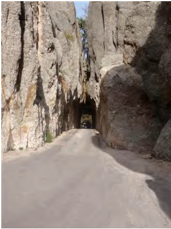
One-Lane Tunnel, Custer State Park, South Dakota
