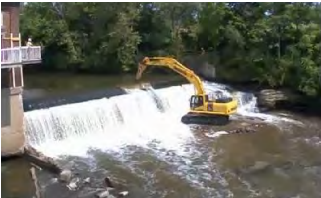
August 13: First cut in the LeFever Dam.
