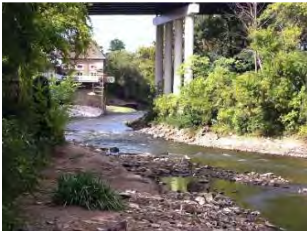
A river runs free! The view of the remains of the LeFever Dam.
