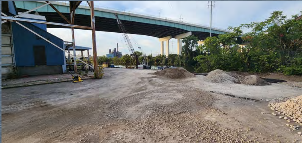
Surface terrain levelling
