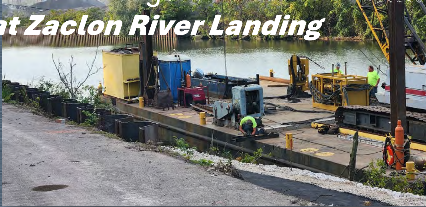
Early shoreline stabilization
