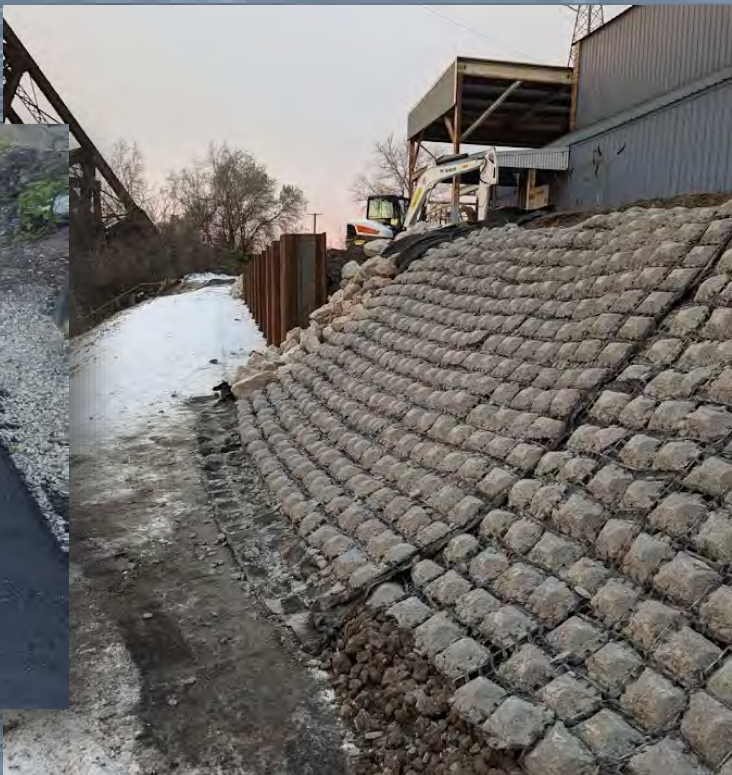
Shoreline remediation & encasement project
